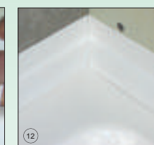
12 Ensure Sealux-N fuses across joints inside strips
