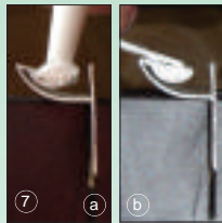
7 (a) lay Sealux-N in strip (b) level Sealux-N in strip
