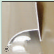
10 Rotate strip into position over ledge
