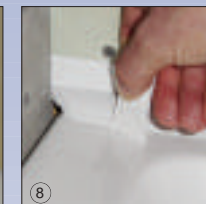
8 Remove excess Sealux-N off ledge if any
