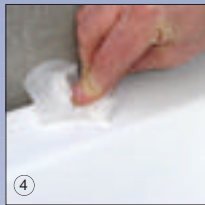
4 Clean ledge using Sealux alcohol/meths wipes
