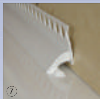
7 Lay strip over joint fusing silicones
