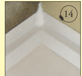
14 Fill notch with Sealux-N as shown
