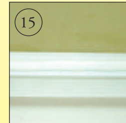
15 Lay Sealux-N bead across strip upstand
