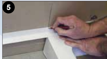
4 Remove saw cut frays. Dry fit strips. Ensure mitre cuts meet. Mark and cut strip end points.
