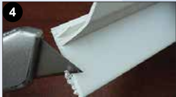
4 Remove saw cut frays. Dry fit strips. Ensure mitre cuts meet. Mark and cut strip end points.
