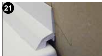
16 Strips may be adjusted before Sealux-N cures to ensure mitre joints match. Flush up Sealux-N at strip ends and fix end caps if required.
