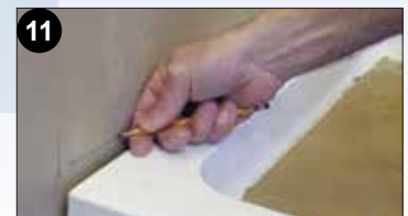
9 Using a strip off-cut in the fitted position, apply 4 marks to each side wall and ledge to define the position for sealant on the wall and the strip outer edge on the ledge. Draw a line through the marks applied on the walls.
