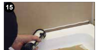
12 Lay a line of Sealux-N on the ledge just inside the 4 marks defining the strip outer edge position. Lay a 4mm (light) line of Sealux-N on the wall over the line applied through the 4 wall marks.
