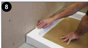
8 Wipe the ledge with alcohol wipes.
