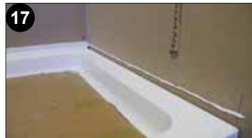
14 Strips may be adjusted before Sealux-N cures to ensure mitre joints match. Flush up Sealux-N at strip ends and fix end caps if required.
