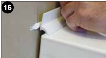
14 Strips may be adjusted before Sealux-N cures to ensure mitre joints match. Flush up Sealux-N at strip ends and fix end caps if required.
