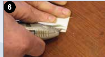
6 If the strip outer edge does not sit on ledge, tear off the removable inner leg.
