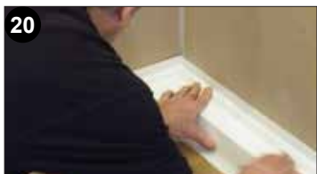
16 Strips may be adjusted before Sealux-N cures to ensure mitre joints match. Flush up Sealux-N at strip ends and fix end caps if required.
