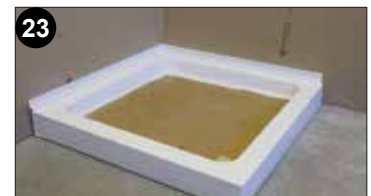
17 Remove any excess Sealux-N on the ledge with spatula. Give the strip and ledge a final wipe. Installation now ready for waterproofing.
