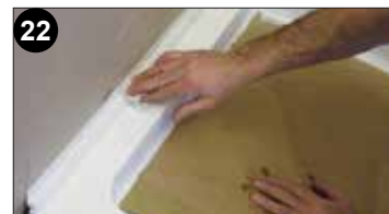
17 Remove any excess Sealux-N on the ledge with spatula. Give the strip and ledge a final wipe. Installation now ready for waterproofing.
