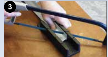
3 Mitre cut all strips being installed.
