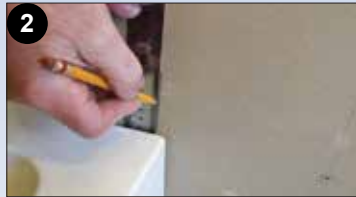
2 Mark the strip end points on walls.
