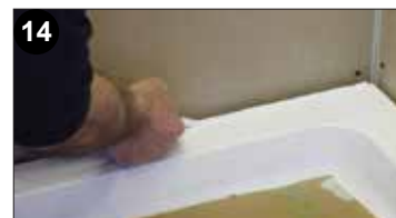
12 Lay a line of Sealux-N on the ledge just inside the 4 marks defining the strip outer edge position. Lay a 4mm (light) line of Sealux-N on the wall over the line applied through the 4 wall marks.
